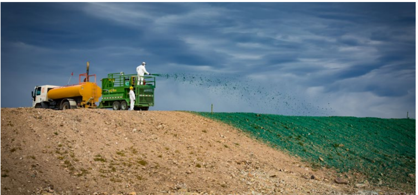
Hydroseeding for reclamation of waste rock dumps at Manantial Espejo.
