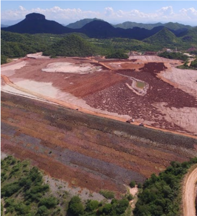
Alamo Dorado Tailings Dry Stack: Before
