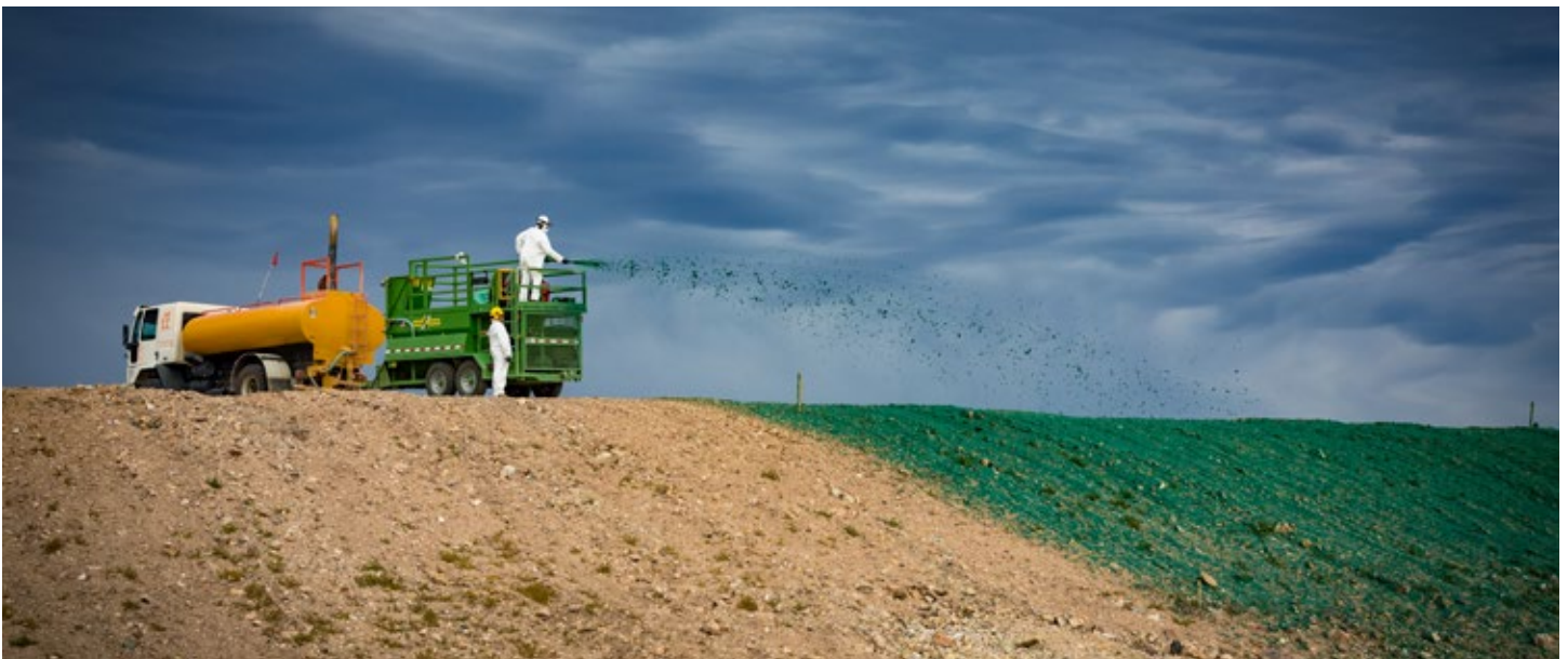
Hydroseeding for reclamation of waste rock dumps at Manantial Espejo.
